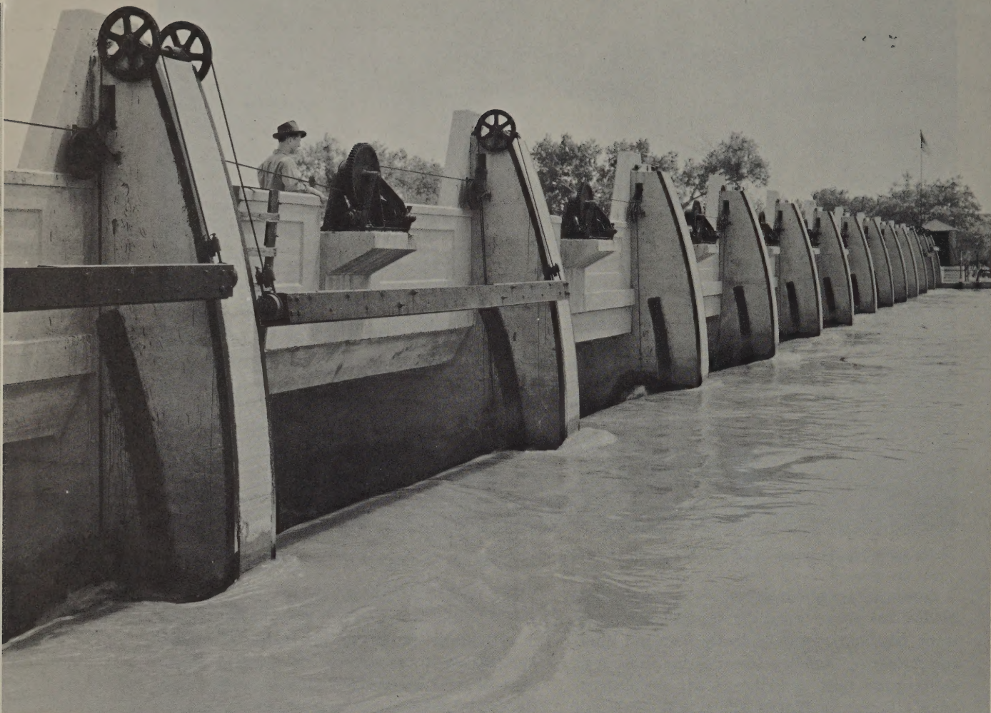
Diversion dams, such as this one at Mesilla, channel the water so necessary for irrigation to nearby farm land.
